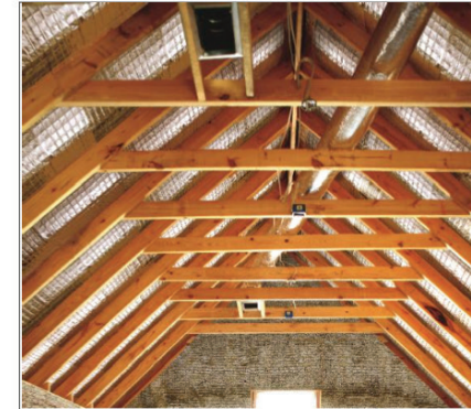
Example installation in a new construction application where the radiant barrier is pre-laminated to the roof decking
